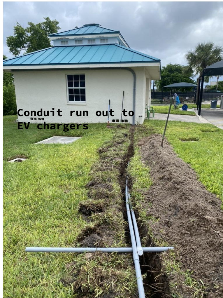
Subpanel And Conduit Out to EV chargers
