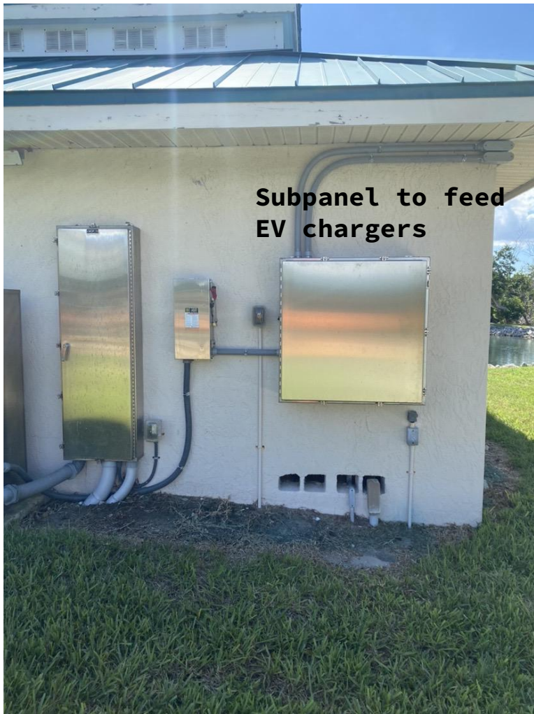
Subpanel And Conduit Out to EV chargers
